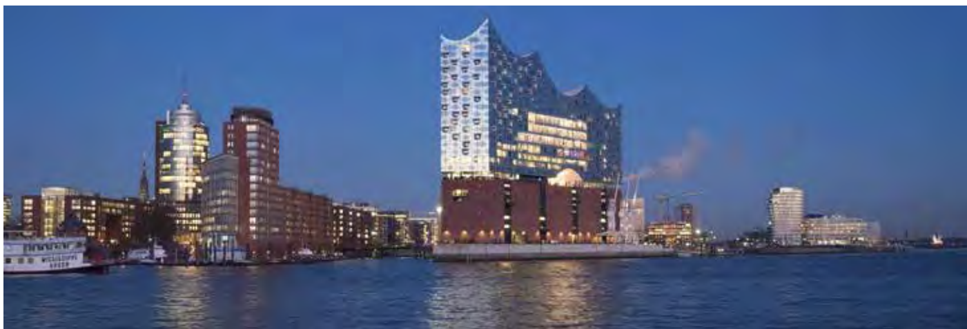
Foto ENGIE Refrigeration: Quiet as a whisper water-cooled chillers at the Elbphilharmonie
